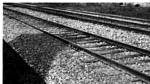
Typical Stone Ballasted Track
