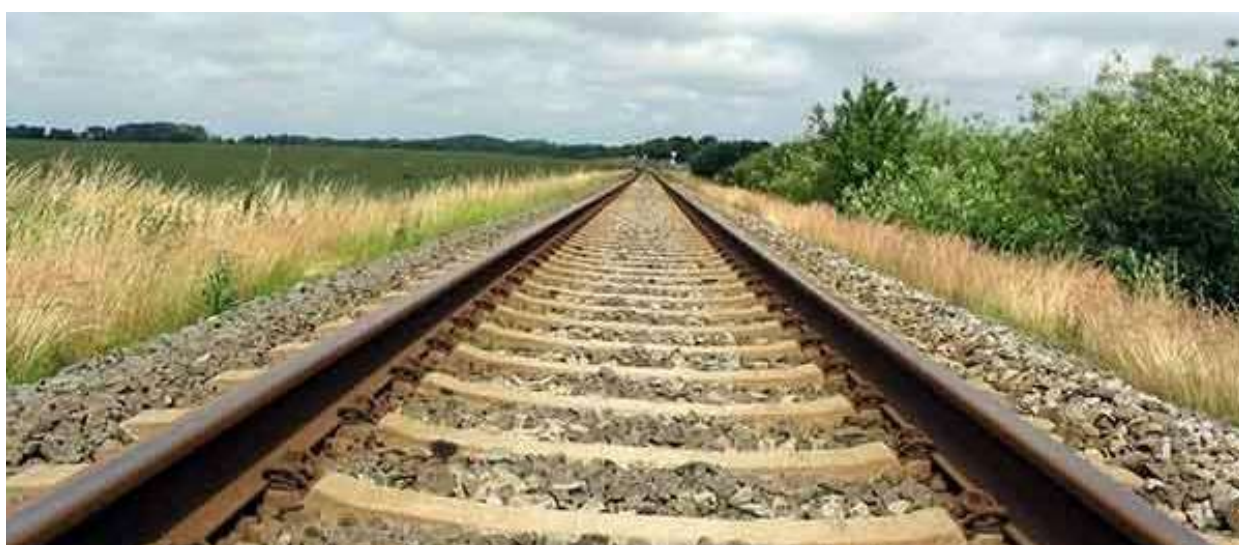
Typical ballast application, with sleepers and sleeper-ends exposed
