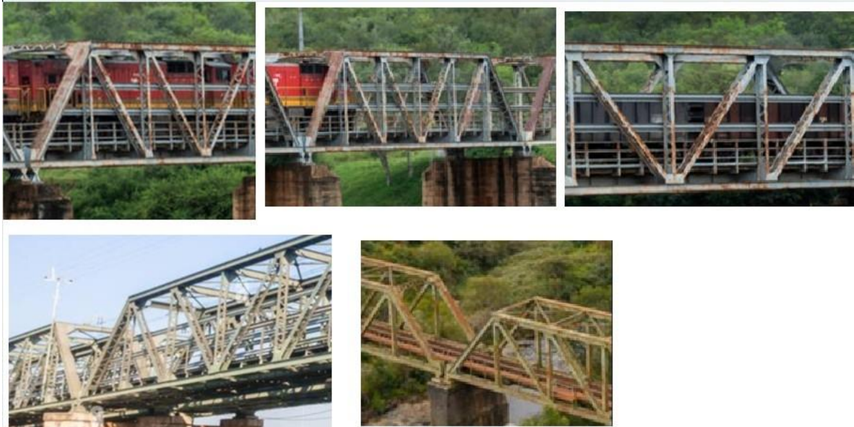
Some pictures of SAR trestle bridges.
